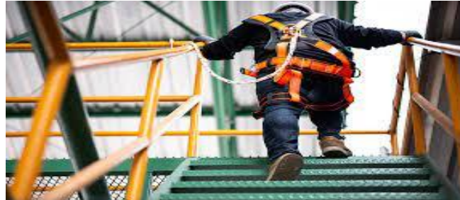
Gambar 1. Hand Railing, Guadrail, Toe Board Sumber: Google Foto
