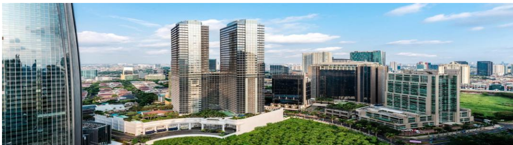
Gambar 3.1 Gedung The Ritz – Carlton Jakarta Mega Kuningan (Sumber: Human Resources The Ritz – Carlton Jakarta 2026)
