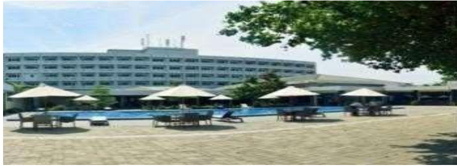
Gambar 3.6 Swimming Pool Sumber: Dokumentasi pribadi
