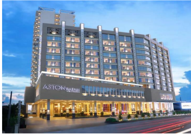
Gambar 1. Aston Batam Hotel And Residence
