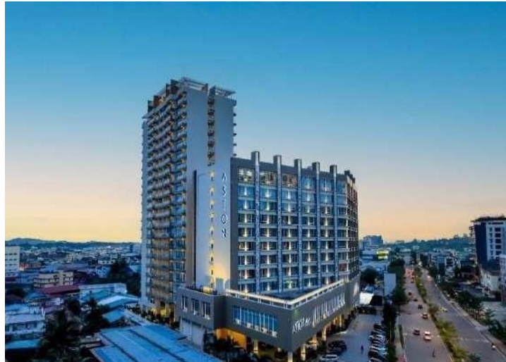
Gambar 3. Aston Batam Hotel & Residence
