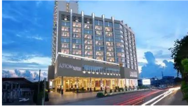
Gambar 3.2 Aston Batam Hotel & Residence
