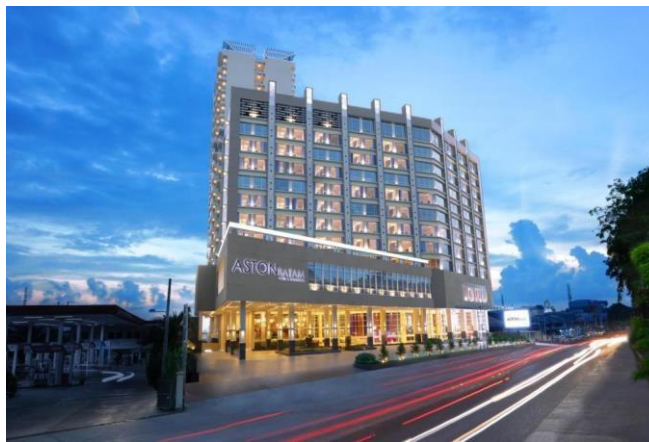
Gambar 2 Aston Batam Hotel & Residence
