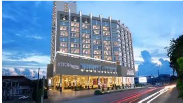
Gambar 3.1 ASTON Batam Hotel & Residence
