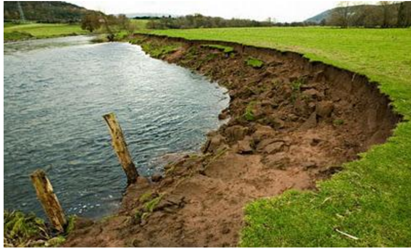
Gambar. II. 1. Erosi Tebing Batang Kapur
