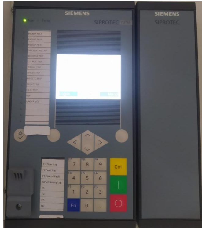
Gambar 3. 20 Relay Differensial SIEMEN SIPROTEC 7UT85
