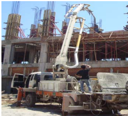
Gambar 9: Concrete Pump
