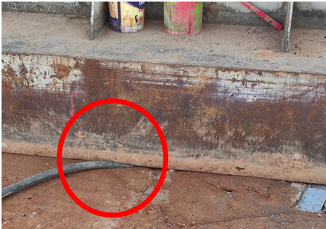
Kabel generator HSPD ( hydraulic static pile driver ) terhimpit alat.
