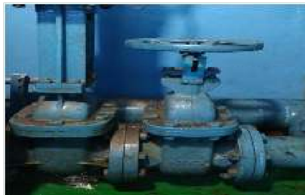
Gambar 4.12 Water Stop Valve
