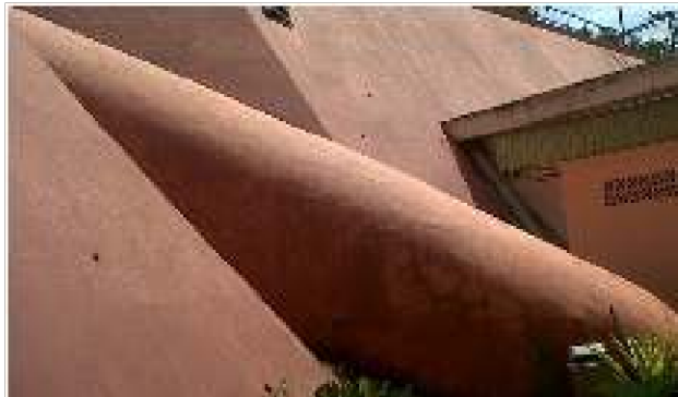
Gambar 2.9 Penstock ( Pipa Pesat )
