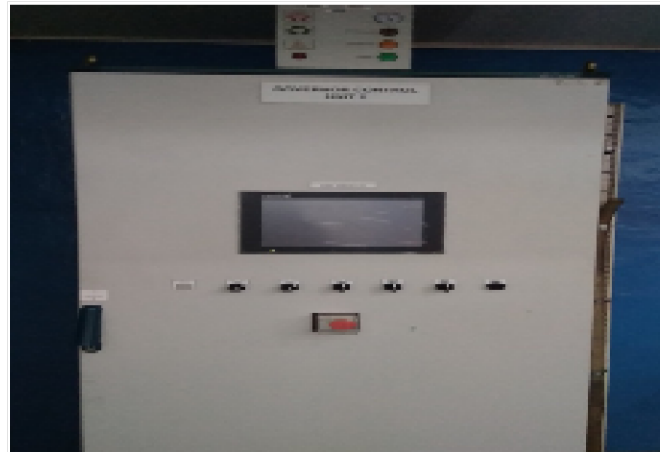
Gambar 2.16 Governor Control PLTA Batang Agam
