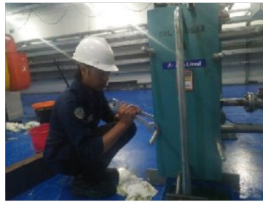
Gambar 4.2.9 penguncian manhole
