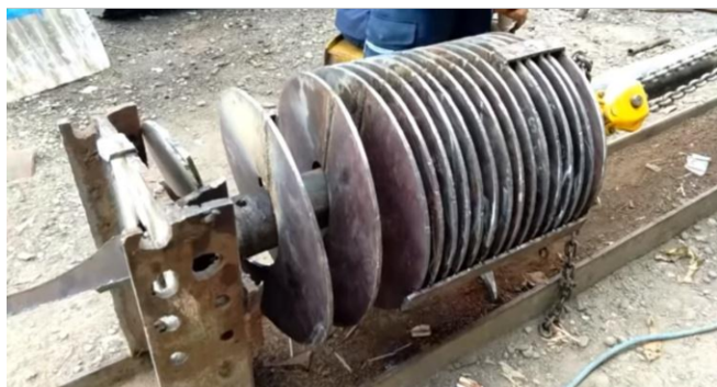
Gambar 4. 6. Pemasangan rantai chain block ke daun screw conveyer
