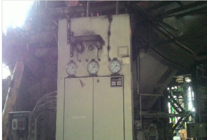
Gambar 3.5 Sistem Pelumasan Roller Mill ( coal mill )
