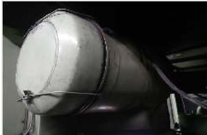
Gambar 4.8 *Air Filter housing*
