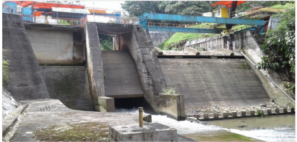
Gambar 1.2. Intake weir PLTA Batang Agam
