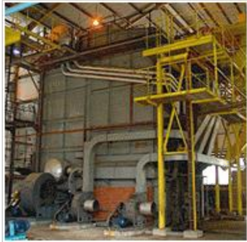
Gambar 23. Vickers Water Tube Boiler
