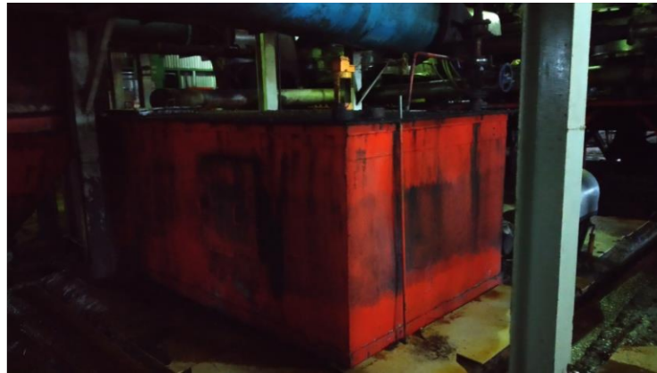
Gambar 2.12 Crude oil tank
