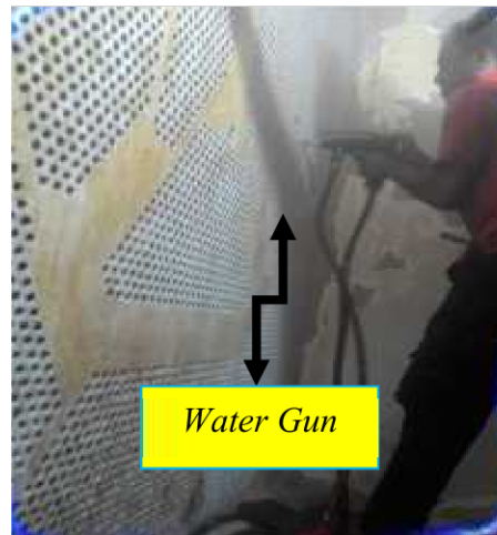
Gambar 12. Perawatan Tube Kondensor
