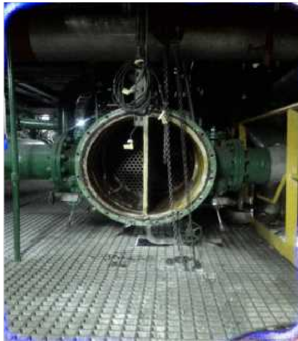
Gambar 13. Perawatan Heat Exchanger
