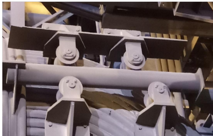
Gambar 4.5 Sliding Sleeve
