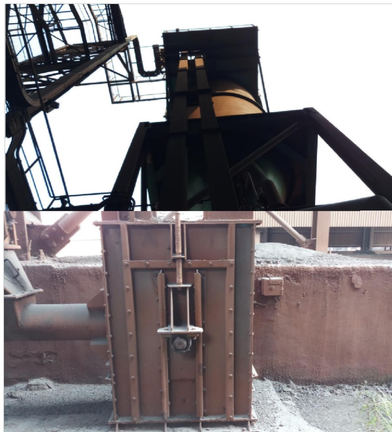
Gambar 4.19 Bucket Elevator
