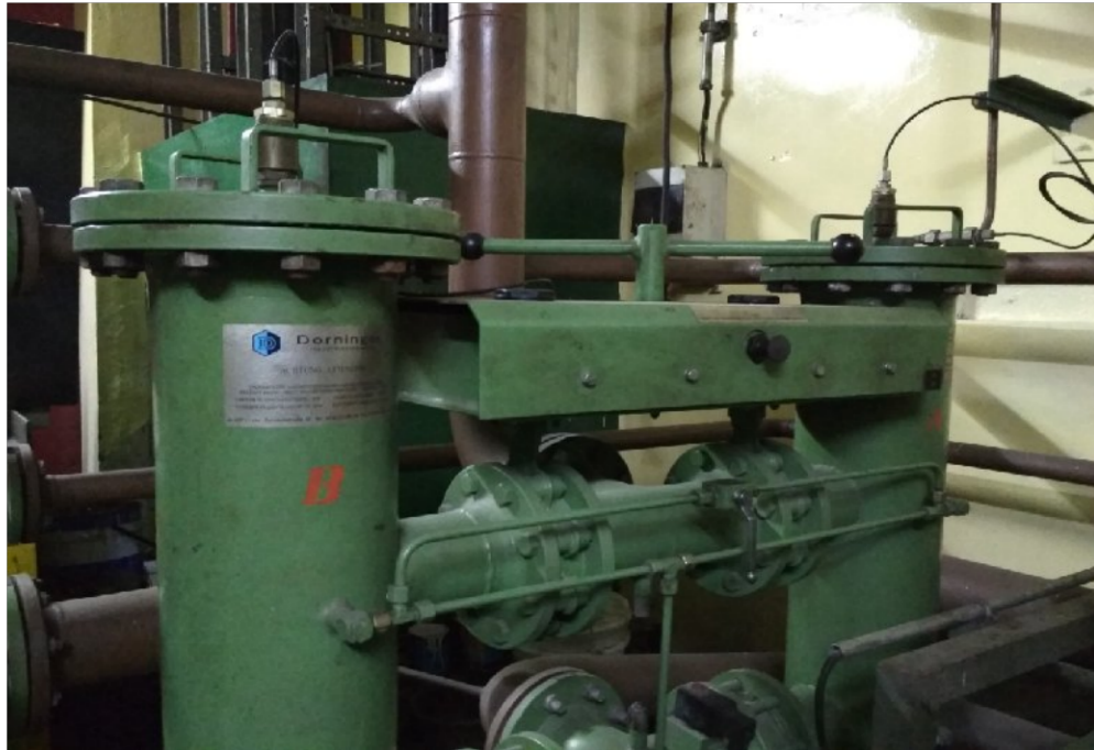
Gambar 5.6 Filter circulation system
