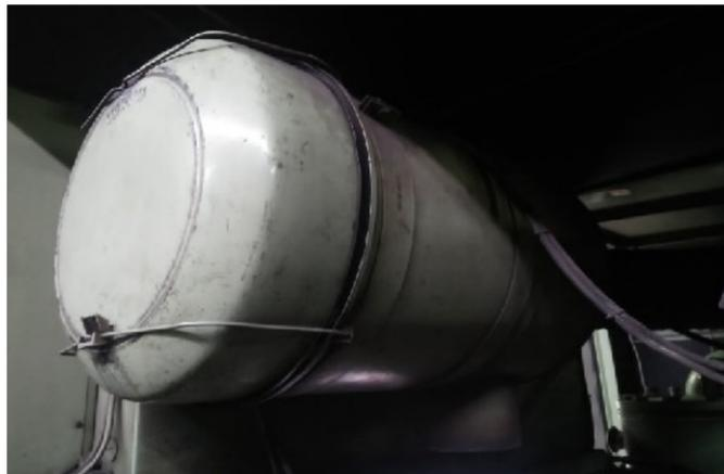
Gambar 4.8 *Air Filter housing*
