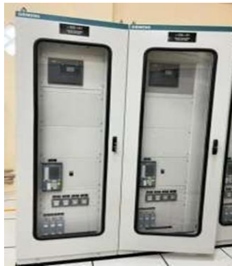
Gambar 2.7 Foto Relay Board
