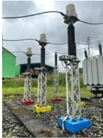
Gambar 2.2 Foto Current Transformer
