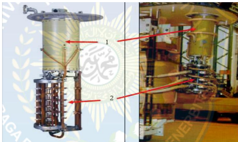
Gambar 2.11 Tap Changer Transformator
