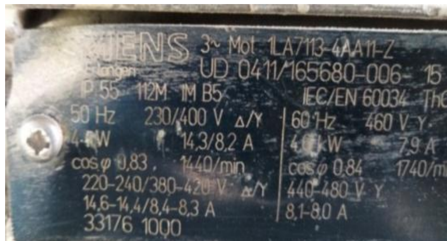
Gambar 4.9 Name Plate Motor S01
