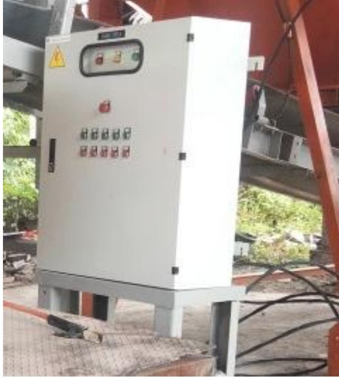
Gambar 4.2 Panel Interlock Brick Transport
