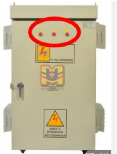
Gambar 12.Lampu indicator
