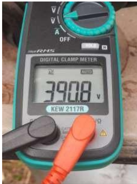
Gambar 4.19 pengukuran tegangan line to line
