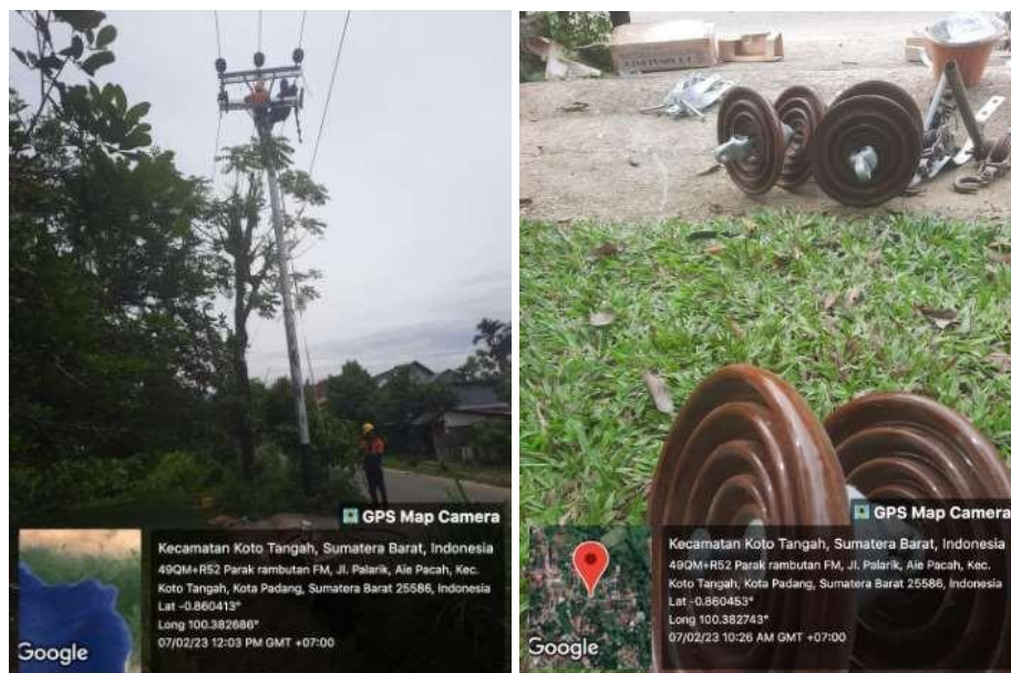
Lampiran 10 Pemasangan Cover FCO (Fuse Cut Out)
