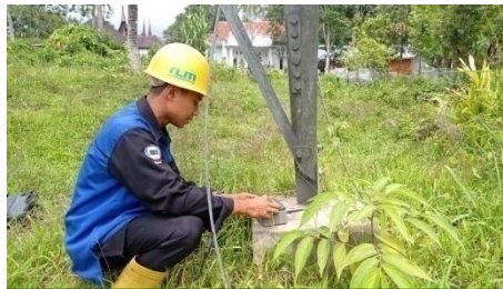
Gambar 5. Pengujian Pentanahan Tower Transmisi
