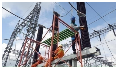
Gambar 18. Proses Cleaning PMT
