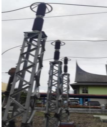
Gambar 9. Lightning Arrester
