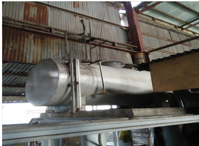
Gambar 24. Water storage Tank Sumber . PT Jaya Sentrikon Indonesia
