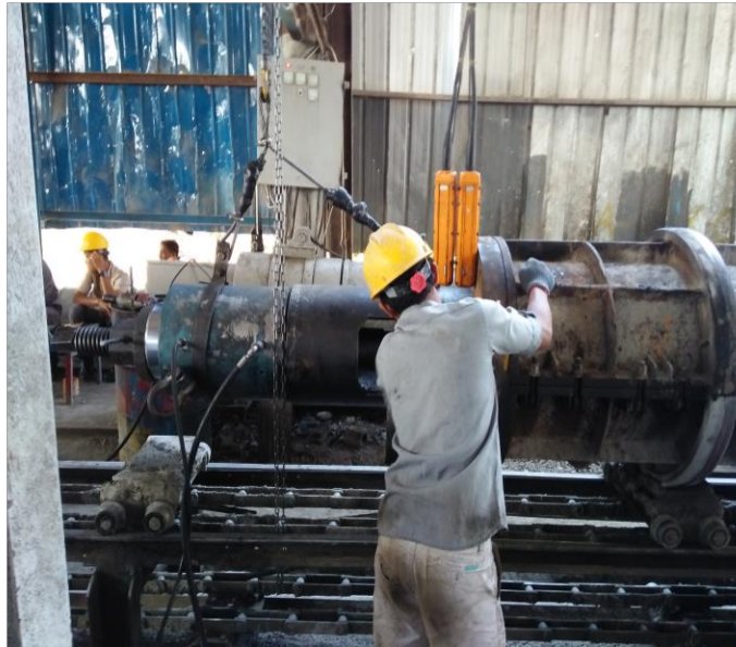
Gambar 13. Tensioning (penarikan besi ) Sumber . PT Jaya Sentrikon Indonesi
