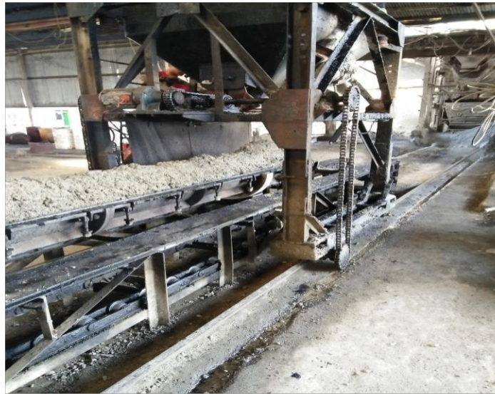
Gambar 12. Placing ( pengecoran beton ) Sumber . PT Jaya Sentrikon Indonesia
