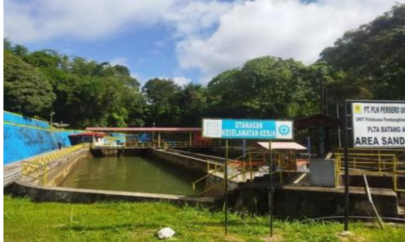
Gambar 6. Sand Trap
