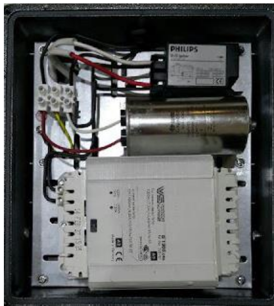
Gambar 29 Bagian-bagian Lampu HPIT
