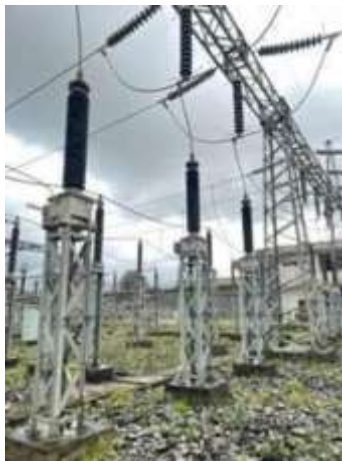
Gambar 2.3 Capasitive Voltage Transformer
