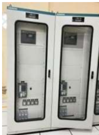
Gambar 2.7 Relay Board
