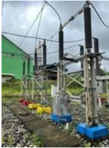
Gambar 2.5 disconnecting switch
