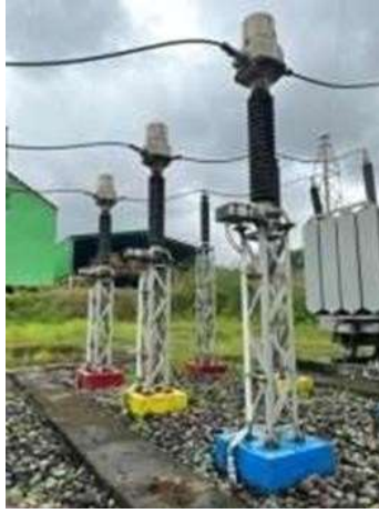
Gambar 2.2 Current Transformer
