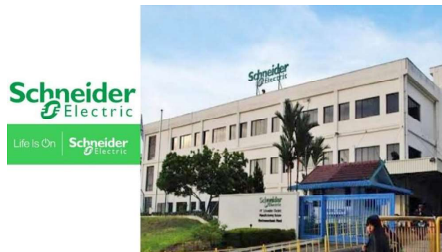
Gambar 1.2 PT Schneider Electric Batam
