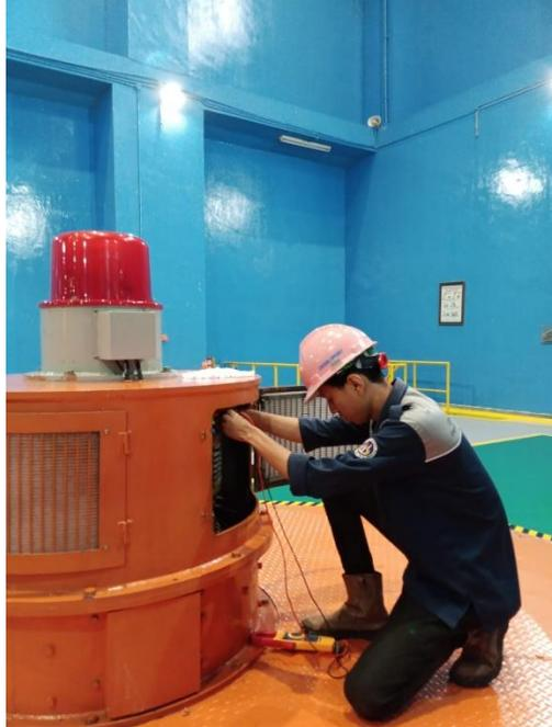
**Gambar 2. 19 Pengecekan *fuse* generator****Foto Kegiatan melakukan pergantian pada lampu generator**
