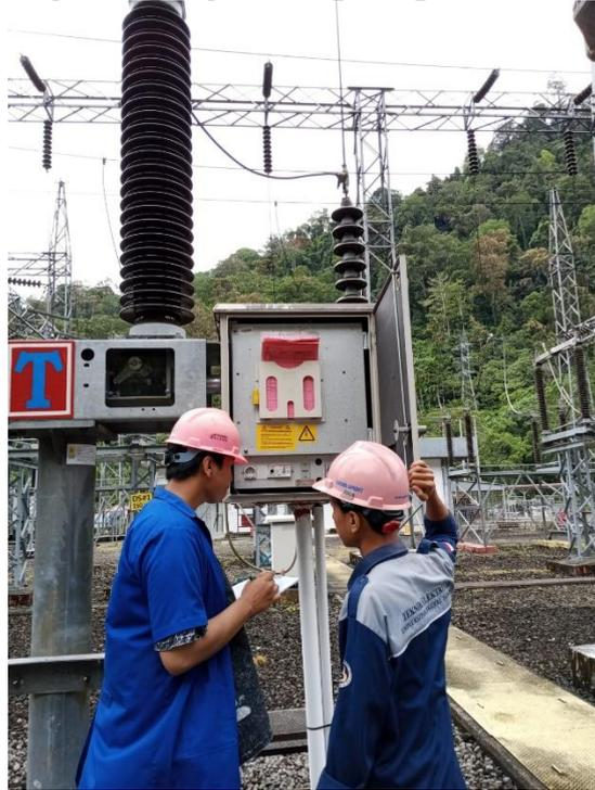
**Gambar 2. 27 Pengecekan panel *DS,PMT,LA***
