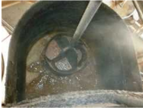
Skimmer Sludge Under Flow
