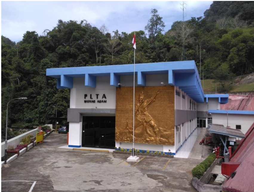
Gambar 2.1 Power House PLTA Batang Agam
