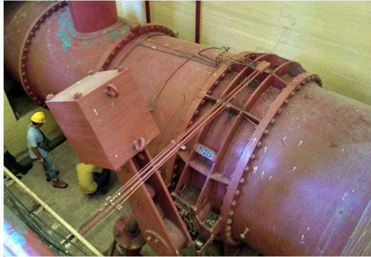
Gambar 2.4 Valve Chamber PLTA Batang Agam
