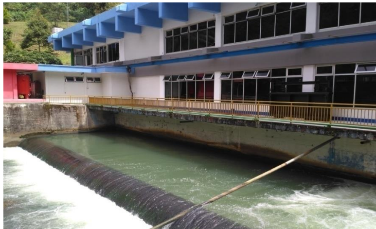
Gambar 2.6 Tail Race PLTA Batang Agam
