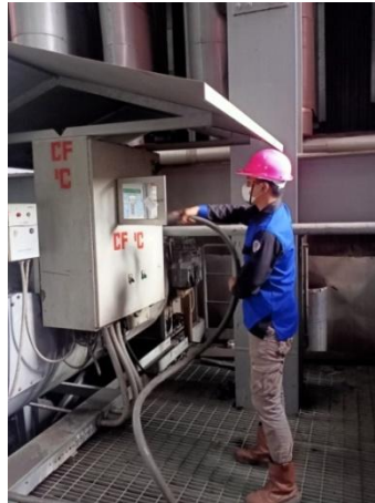
Gambar 3. Proses cleaning panel coal feeder
