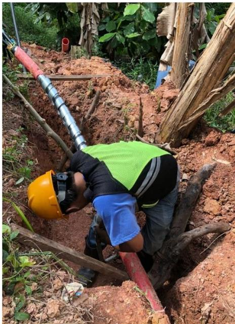
Gambar 2.6 Proses pengupasan selimut aluminium kabel SKTM
