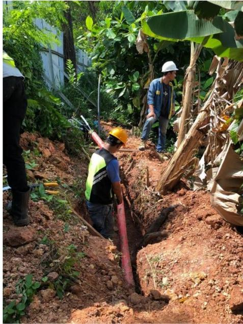
Gambar 2.5 Proses Pengupasan Kabel SKTM
