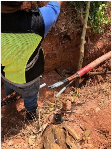
Gambar 2.11 Proses pemberian tanda titik jointing SKTM
