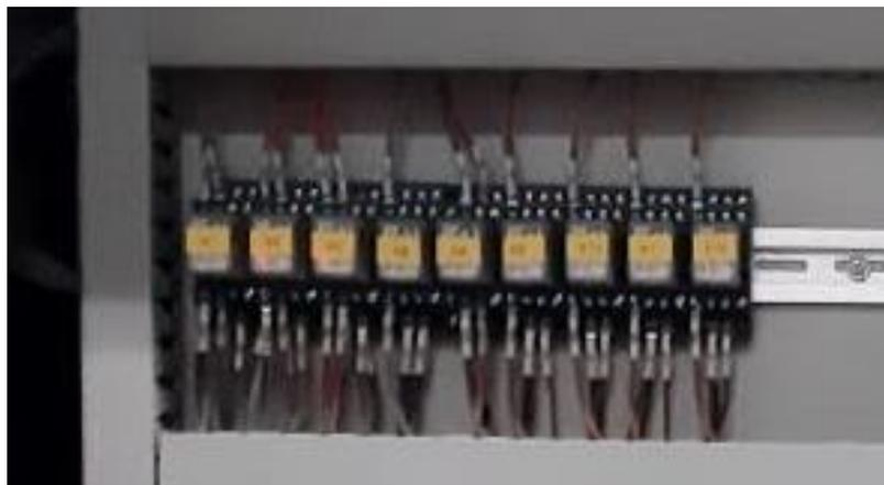
Gambar 3. 12 *Auxiliary Relay*
