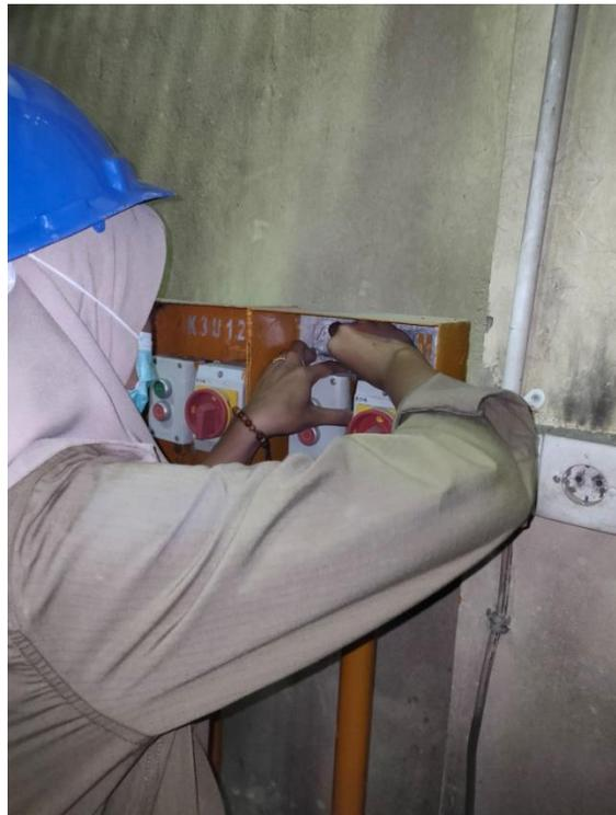
3. Pengecekan oil temperature dan winding temperature pada trafo area LC 20, LC 21.
