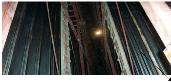
Gambar 6. Collecting Plate ESP
