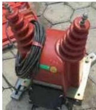
Gambar 4.2 Trafo Tegangan (PT)
