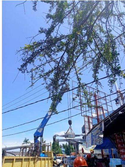
Gambar 4. 11 Proses Penurunan PMT LBSM
