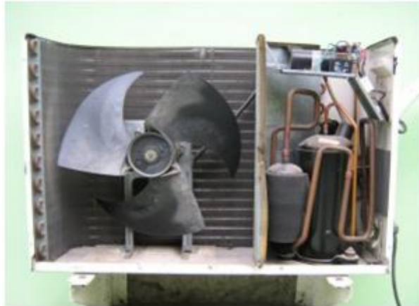
Gambar 2.5 Kondensor
