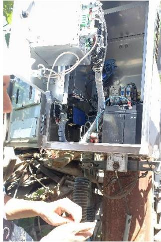
*Gambar 3. 17 Penggantian Modem Sanxing 4G di LBS Truntum*
