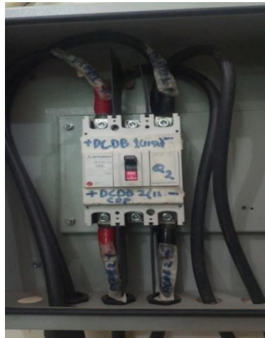
Gambar 4.8 Panel Change Over Switch
