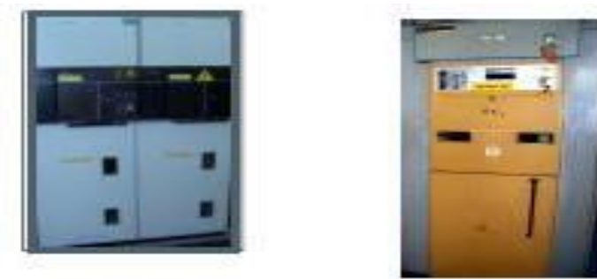
Gambar 4.2 Load Break Switch [9]
