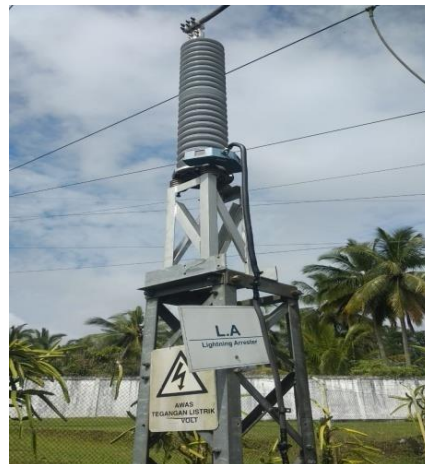
Gambar 3.13 Lightning Arrester
