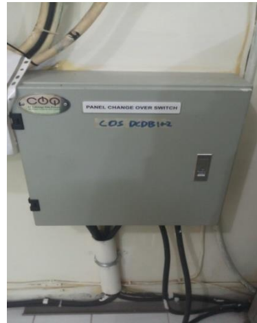
Gambar 4.8 Panel Change Over Switch
