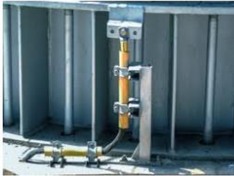
Gambar 12 Grounding generator
