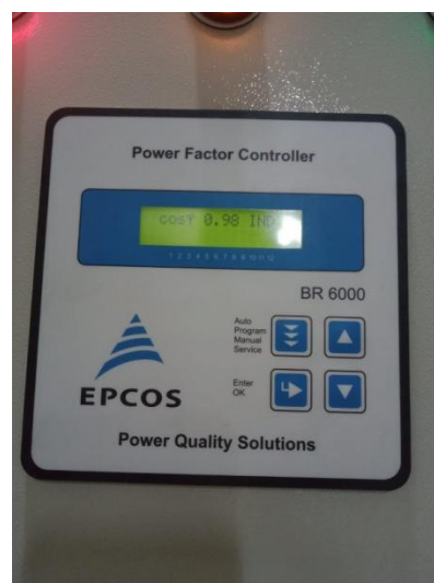
Gambar 37. Reactive Power Regulator
