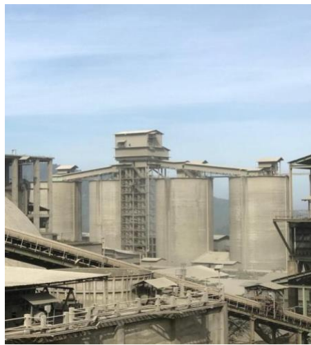
Gambar 12. Silo Cement Mill
