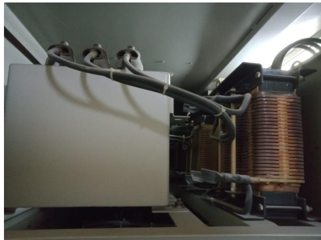
Gambar 41. Current Transformer
