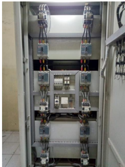
Gambar 50. Kapasitor bank panel per step
