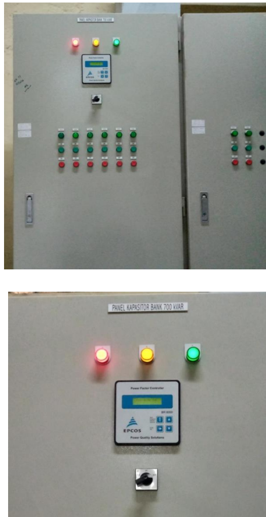
Gambar 45. Panel kapasitor bank 5U1Q32Q6
