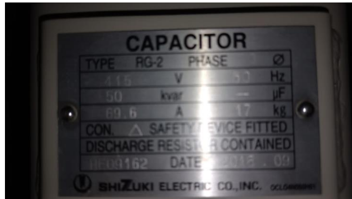
Gambar 46. Kapasitor bank shizuki
