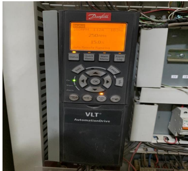
Gambar 29. Variable Speed Drive (VSD) VLT Automation Drive FC 301/302
