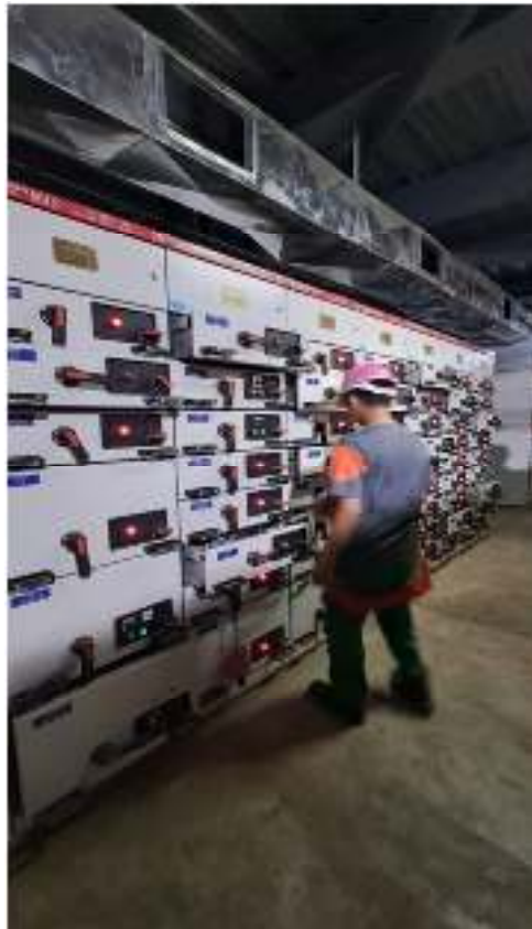
PM (Preventive Maintenance) cleaning Breaker
