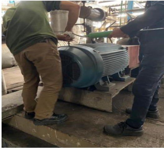
Gambar 2. 26 Proses Pemberian Grease motor
