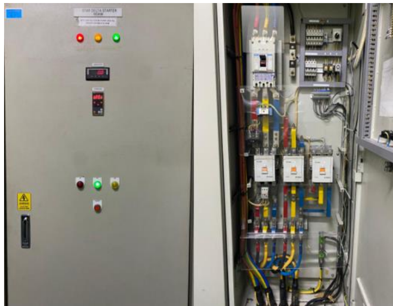
Gambar 2. 7 Panel Star Delta Starter 185 kW
