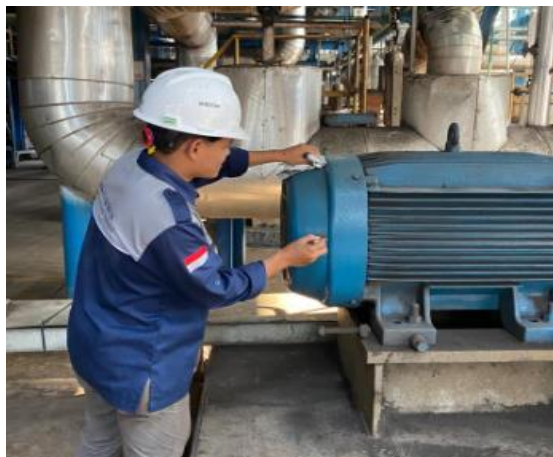
Gambar 2. 29 Cleaning Motor DCB Area
